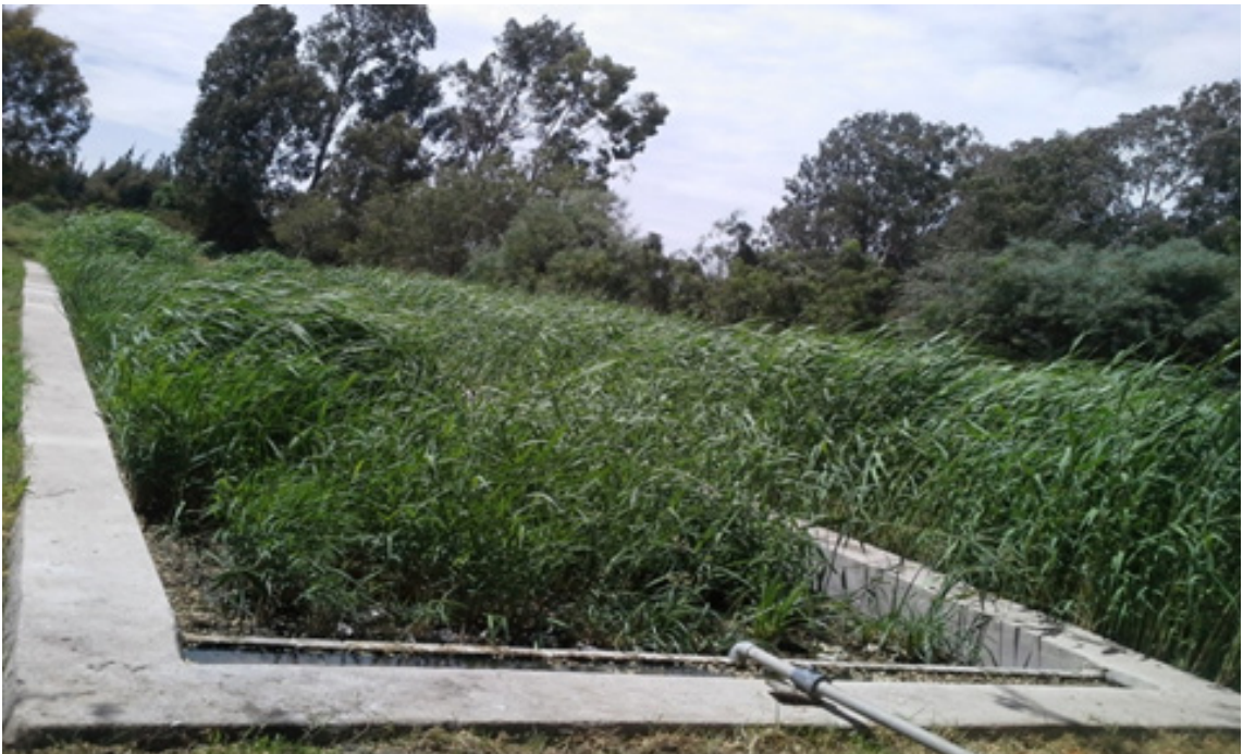
Figure 68: Constructed wetland using phragmites ( P. karka ) for treating tannery industrial waste waters at Mojo, Ethiopia
