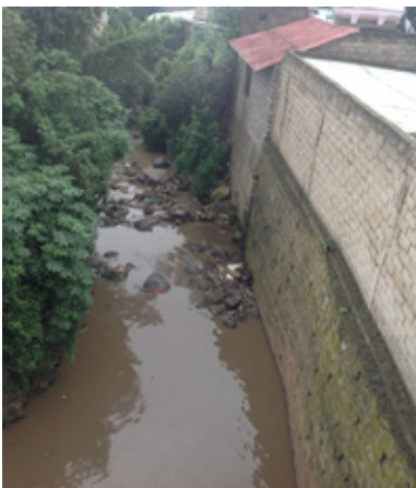
Figure 17: Discharge of wastewater from Kokobe Tsebah School to Kebena river
