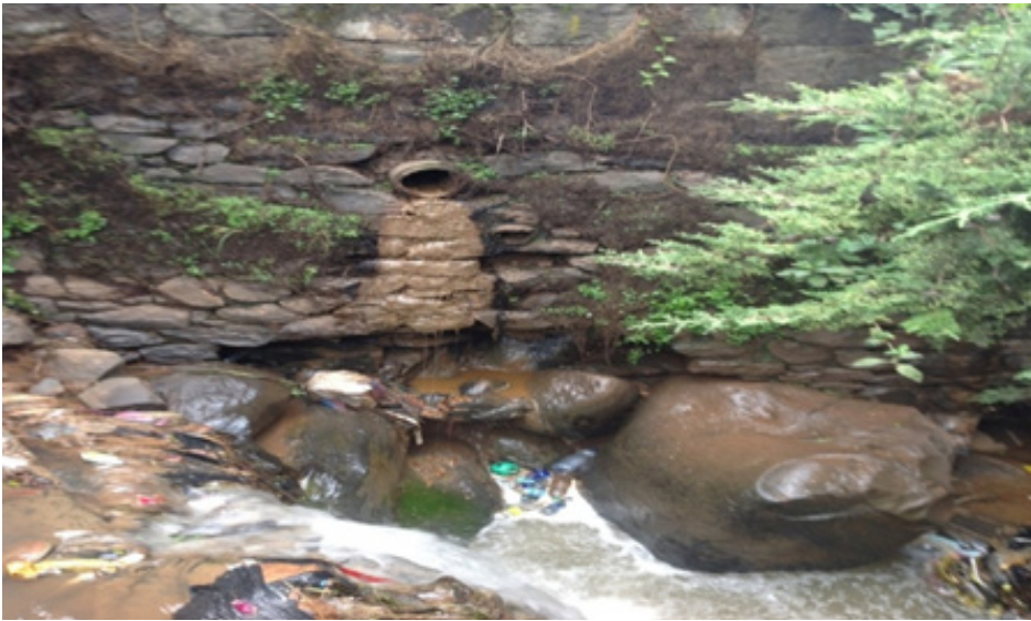
Figure 20: Direct connection of toilets by Shager Park, police station and Hagbes company along Kurtume river
