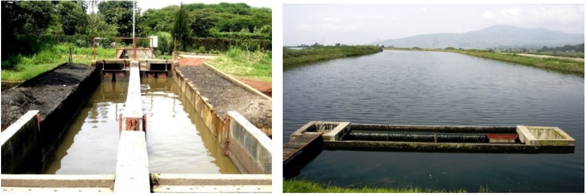
Figure 10: Kality wastewater treatment plant
